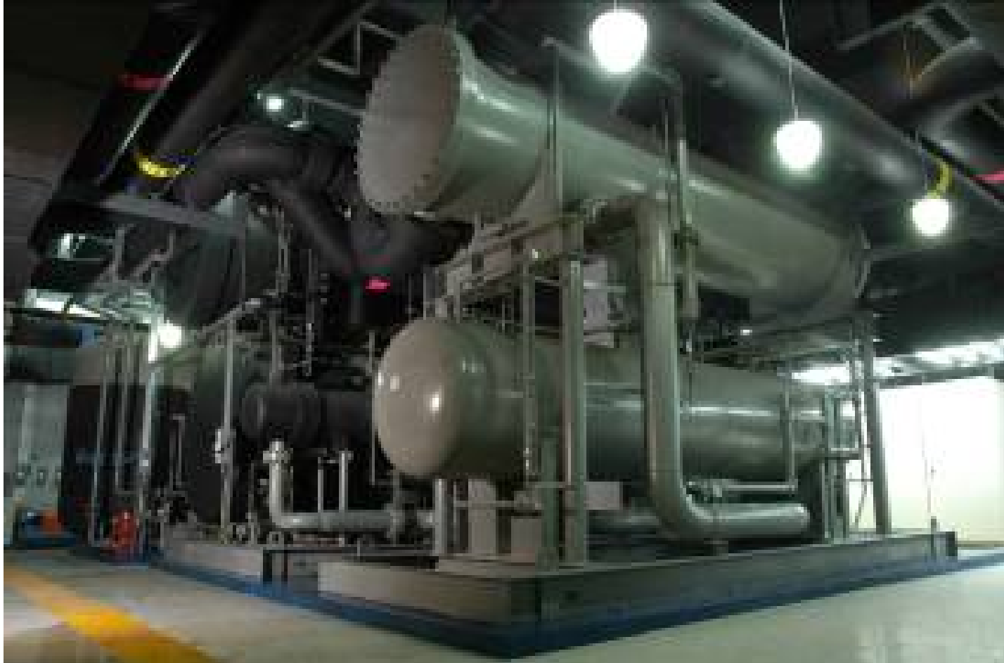
Double evaporator chiller
