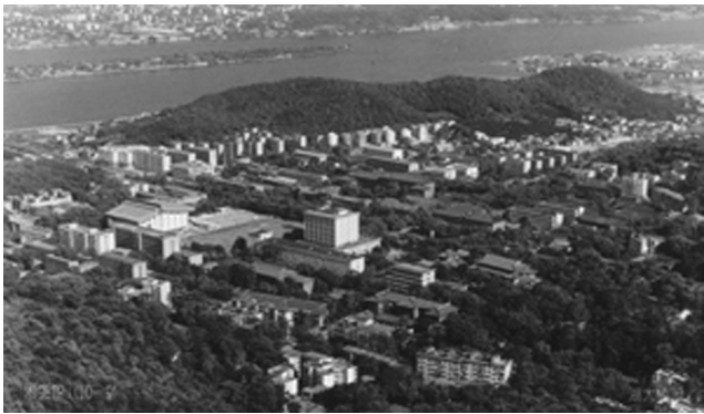
Fig. 1. General view of investigated university and ambient environment.
